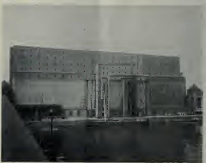
194 x 127 ft. extension to the elevators of the Montreal Harbor Commission.
